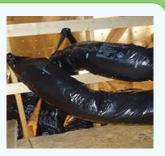
Ducts should not be pinched or constricted to avoid restriced air flow.
