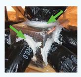
Junction boxes and duct connections should be sealed with mastic.
