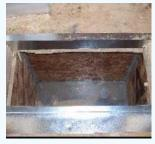
Seal seams in framed wall returns. Note: framed supply ducts are not permitted.
