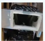
Boots should be sealed at all connecto the interior finish.
