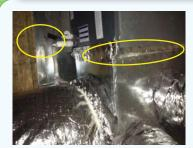
Seal all connections in mechanical cabinet including refrigerant lines, condensate tion points including lines, plenum connections and other seams and holes.
