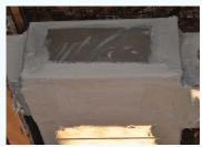
Trunk ducts should be sealed at all joints, seams, and corners with mastic.
